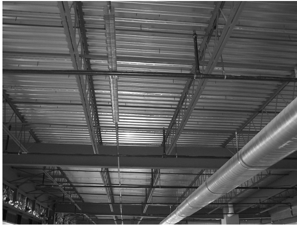
Figure 8-3 Steel-Pan Floor Construction
