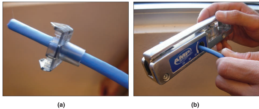
FIGURE 2-14 (a) Placing a bend-limiting strain-relief boot on the cable and (b) stripping off 3 inches of jacket from the UTP cable.
