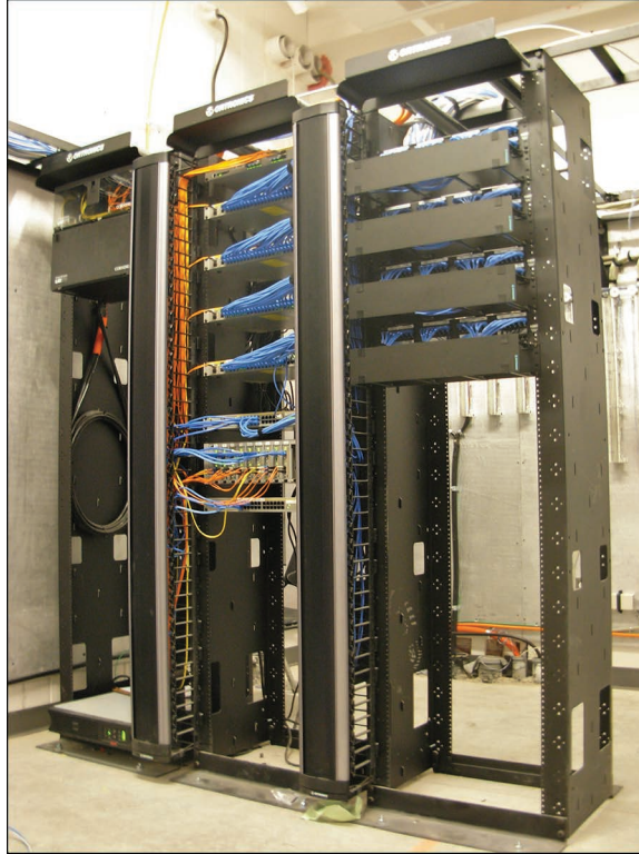
FIGURE 2-5 Inside a telecommunications closet.
