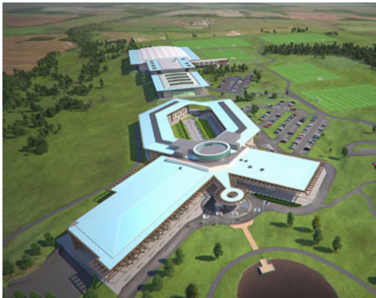
St George's Park under construction: When work is complete, the FA's Burton-upon-Trent site will offer state-of-the-art training and coaching facilities
