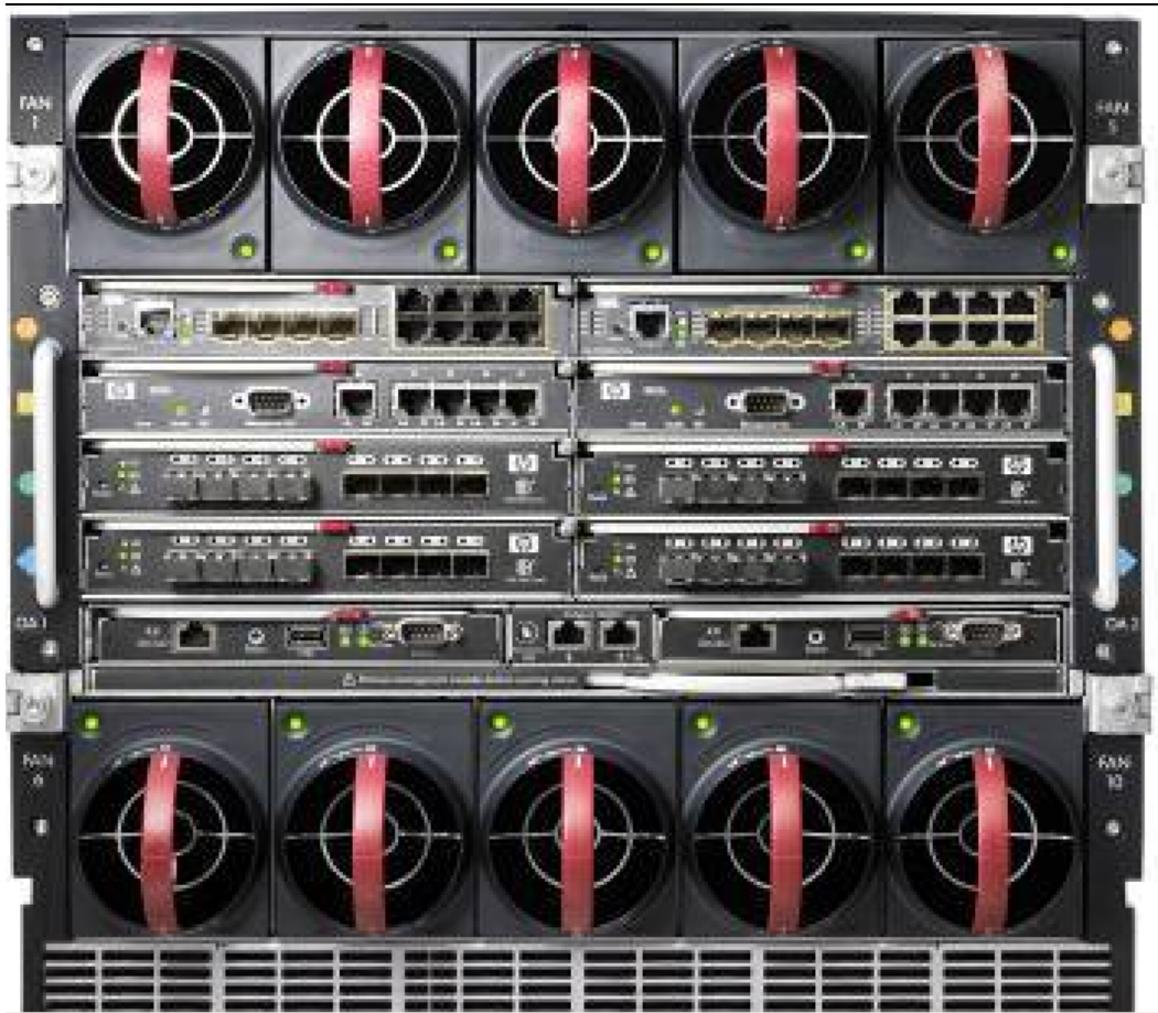
Figure 3-5 HP BladeSystem Rear View
